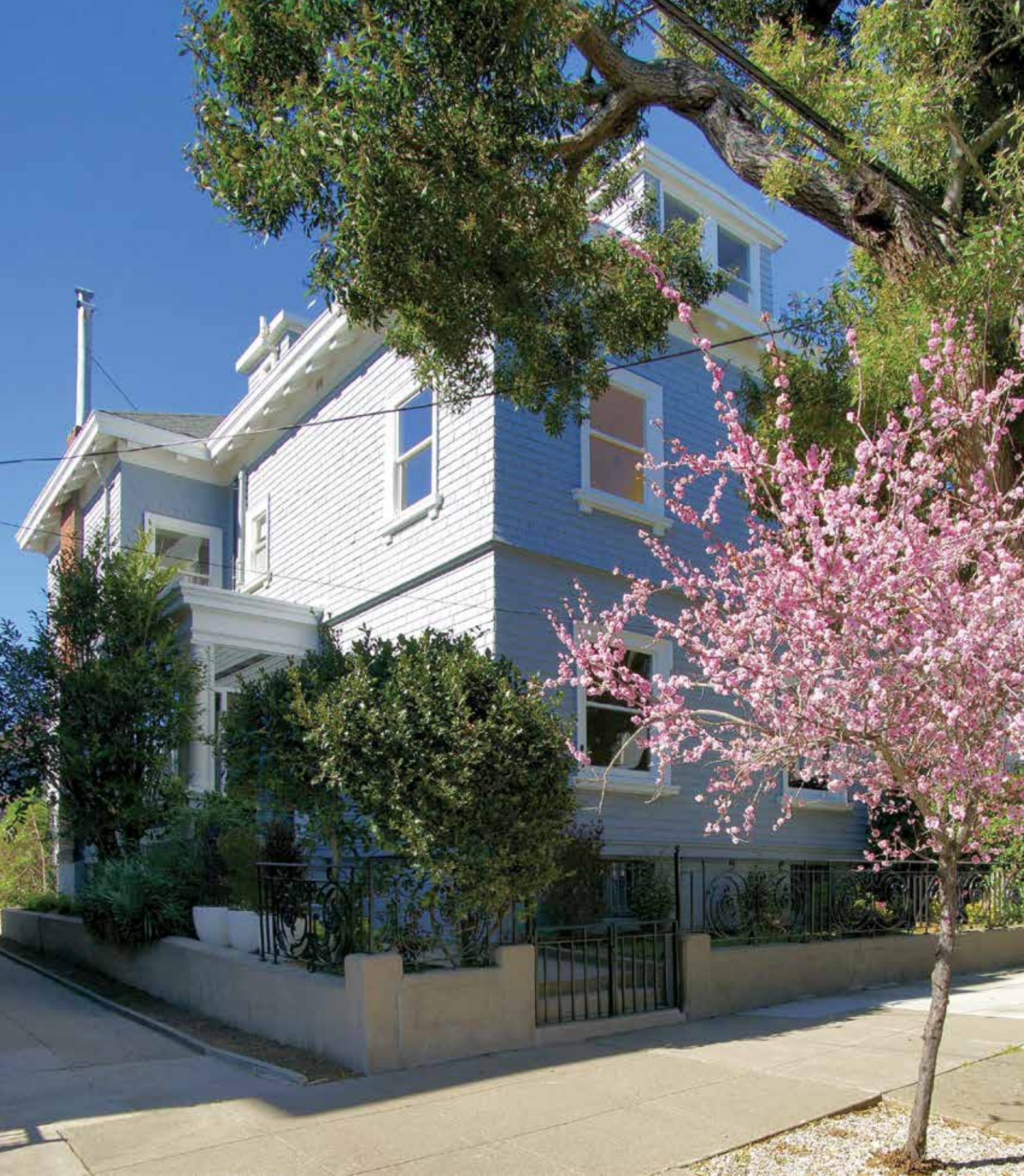
127 5 th AVENUE, SAN FRANCISCO LAKE STREET CORRIDOR EDWARDIAN RESIDENCE
